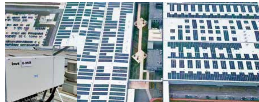
◆.◆MW ENOVATE Motors EV Manufacturing Base PV Plant in Changsha, China (XG◆◆◆KTR XG◆◆KTR)
