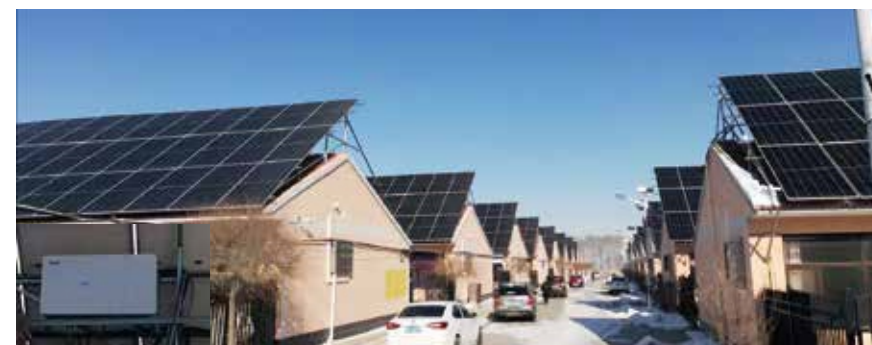
◆◆.◆MW Rooftop PV Plant in Hebei, China (XG◆◆◆KTR .XG◆◆KTR)
