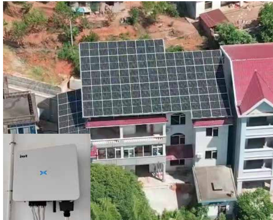
4kW Solar System in Jiangxi, China (XG4KTR)
